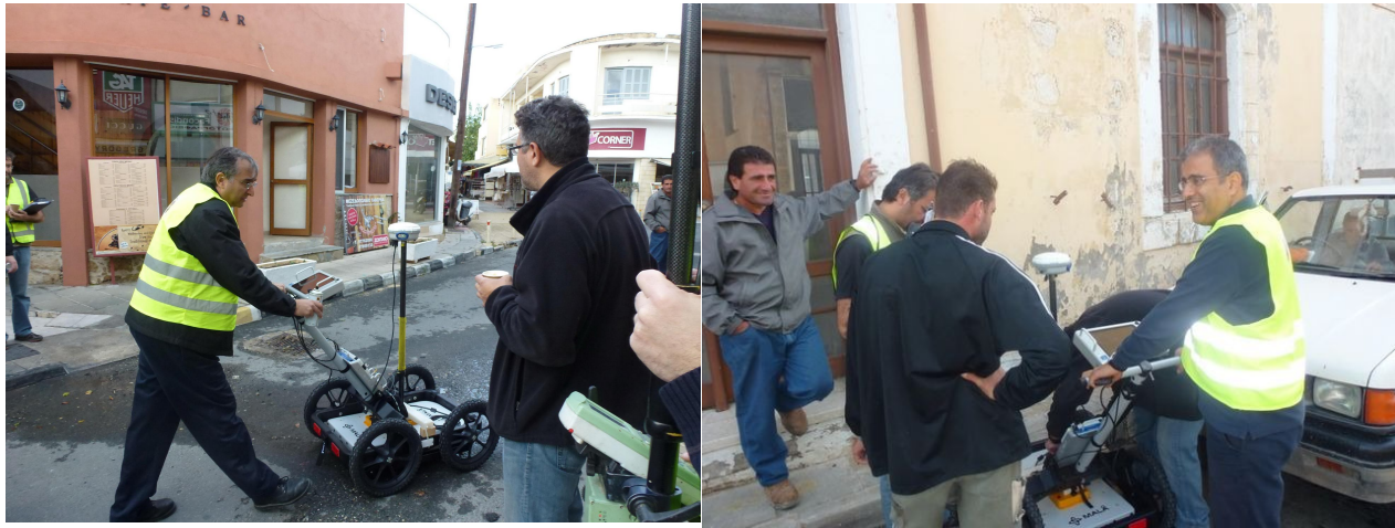
Figure 2.a & b - Geo-radar Scanning of the Paphos water utility network
