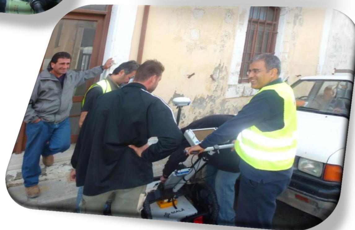
Figure 1.a & b Geo-radar Scanning of the Paphos water utility network
